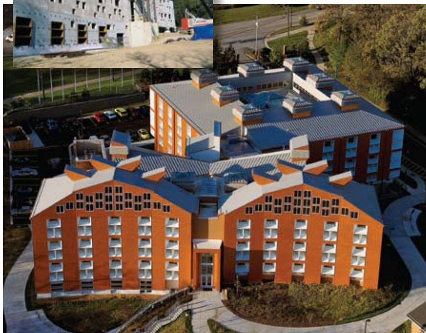
The new academic center features three building segments clad with insulated precast concrete panels. Included are the library (square building at top), central academic wing (narrow shape in middle), and space for the Division of Art, Design & Architecture (sloped-roof structures in foreground).
